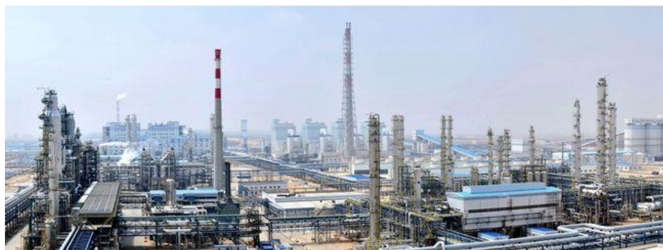
Figure 1. The chemical manufacturing site (Photo courtesy of Shaanxi Yanchang Zhongmei Yulin Energy & Chemical Plant)
