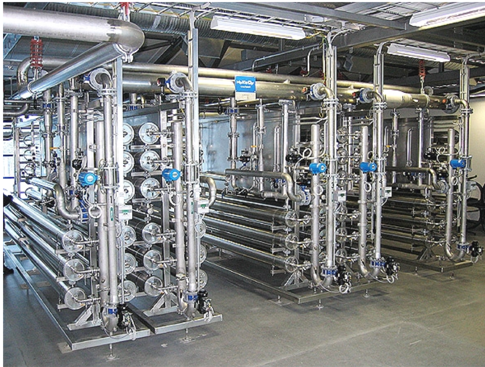
Photo courtesy of HyXo and Kymenlaakso Water Ltd.
