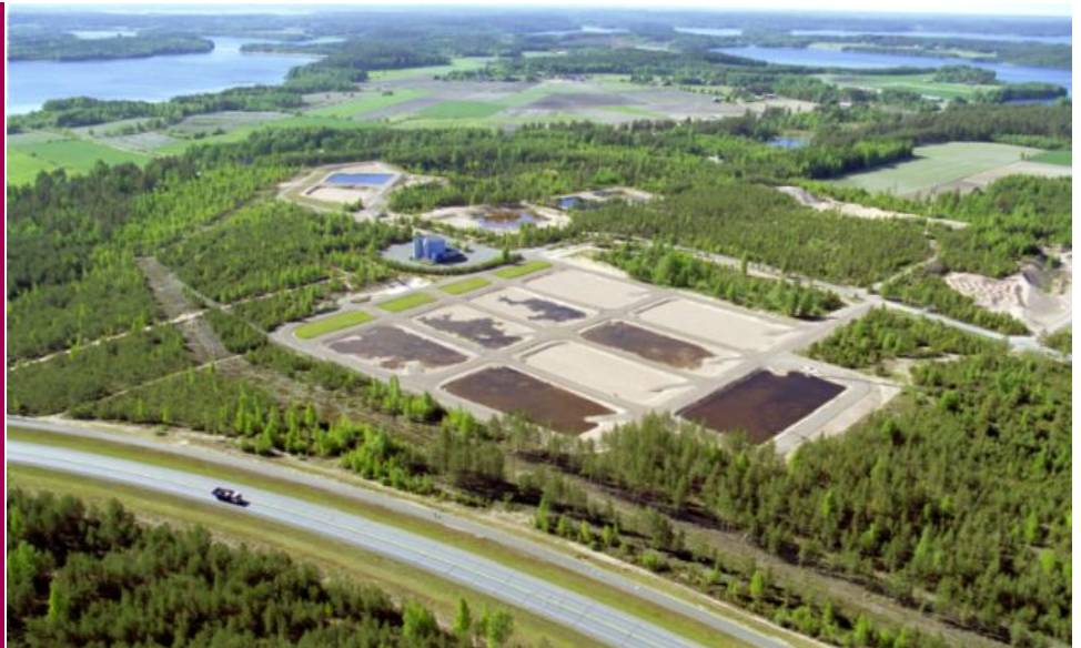
An aerial view of the Kuivala water treatment plant in southern Finland. The plant uses FILMTEC™ XLE reverse osmosis membranes to remove fluoride from drinking water.
