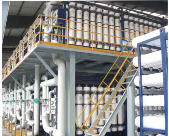
Two-floor arrangement of DuPont™ Ultrafiltration SFP-2860 modules in the Taiyuan facility. (Photo courtesy of Taiyuan Steel Group Co. Ltd.)
