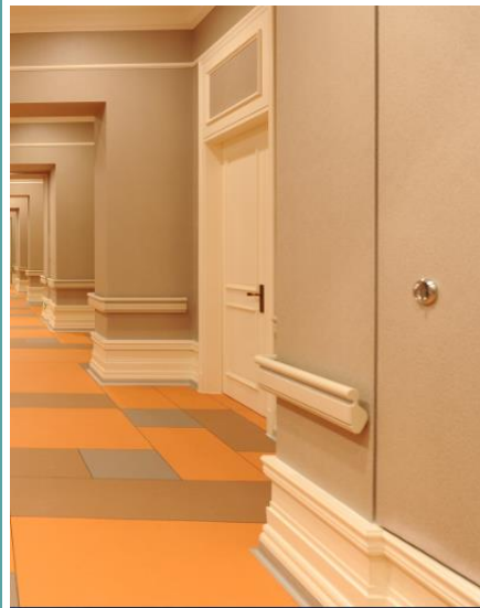
Diagnostic office: fiber-cement plasterboard laminated with Tedlar® wallcovering
