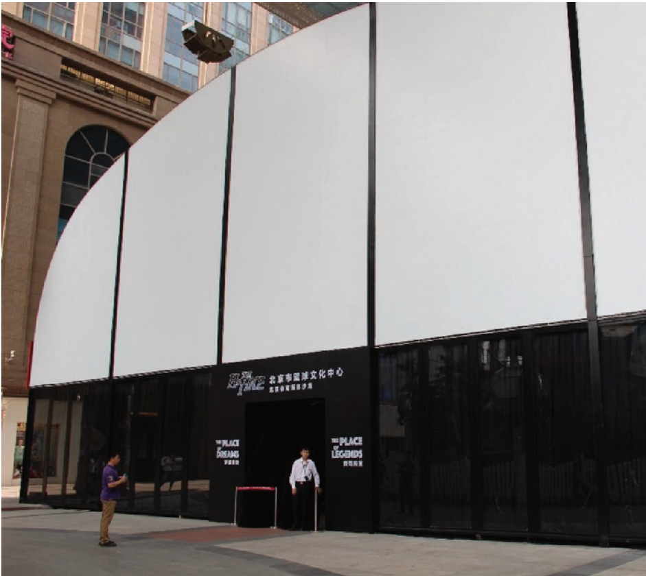
Beijing Urban Basketball Center (China)
