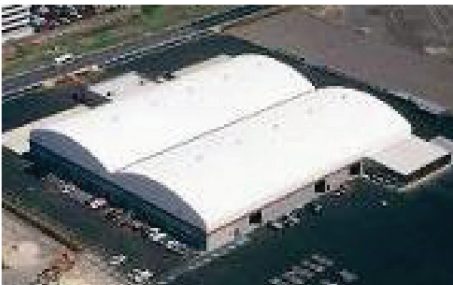
Airport facility (US)
