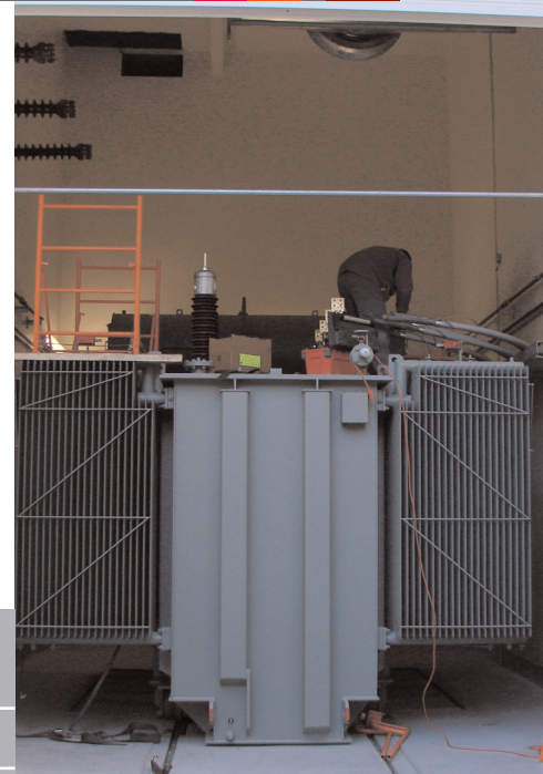
Installation, in the densely populated urban areas of Grenoble, of Pauwels fluid-filled 36 MVA transformer, using a hybrid insulation system based on DuPont™ Nomex® thermal technology.
