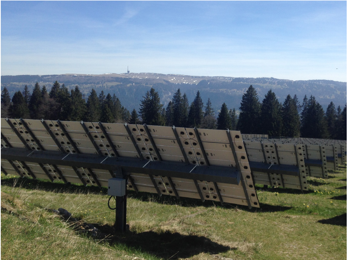
The solar panels at Mont-Soleil face south and are angled at 50° to maximize electricity during the winter months and to help shed snow.
