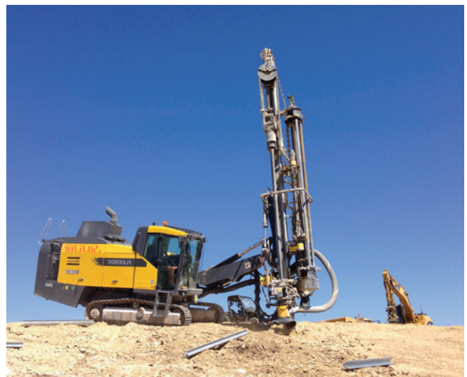
Rock breaker drilling holes for panel substructures
