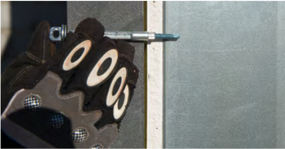
Length of screw into Styrofoam™ Brand Ultra SL insulation board
