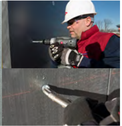
Note: If fastener is not in horizontal position, use a pair of pliers to rotate.
