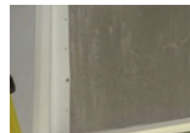
PVC attached to tilt-up wall
