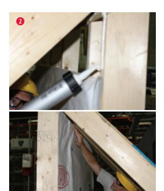
2. Apply DuPont™ Residential Sealant, or recommended sealant, along the top plate and to the remaining 12" of the first and last studs. Install the second layer of the Tyvek® WRB with proper overlap onto the first layer by pressing it into the sealant using firm hand pressure or a J-roller to ensure a good bond between the Tyvek® WRB and the framing.
