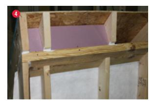
4. Cut  $\frac{1}{2}$ " expanded polystyrene or equivalent foam blocking to fit openings at rafters and install.
