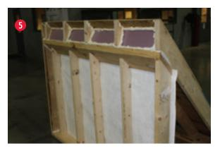
Use **DuPont™ Window & Door Foam** to complete seal around foam blocking.
