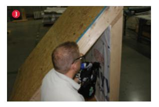
Fasten the DuPont™ Tyvek® WRB to the studs as instructed in the DuPont™ Tyvek® Water-Resistive and Air Barriers Installation Guidelines For Buildings Less Than 5 Stories and Low-Rise Multi-Family Residential Buildings Less Than 6 Stories.
