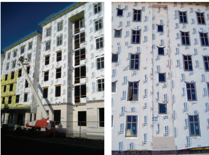
Figure 3. The Ramona Apartment: DuPont™ Tyvek® CommercialWrap® air Barrier was installed over the exterior gypsum board sheathing, with mechanical fasteners.
