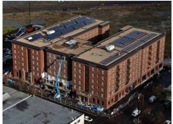
Figure 4. The Ramona Apartments: Brick veneer was installed as exterior cladding.
