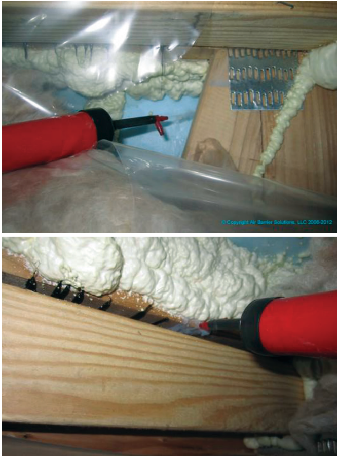
Figure 7. Use of tracer smoke to identify the location and severity of air leakage paths (Source: Ramona Apartments Building Envelope Inspection Report)
